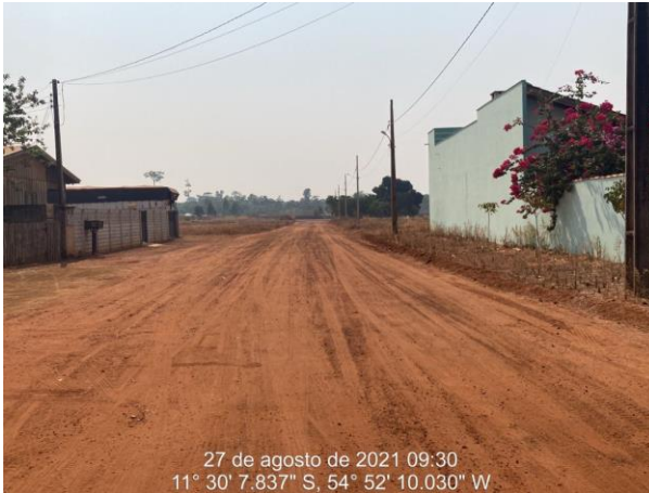
Figura 01: Rua Campos Sales/MT423.
